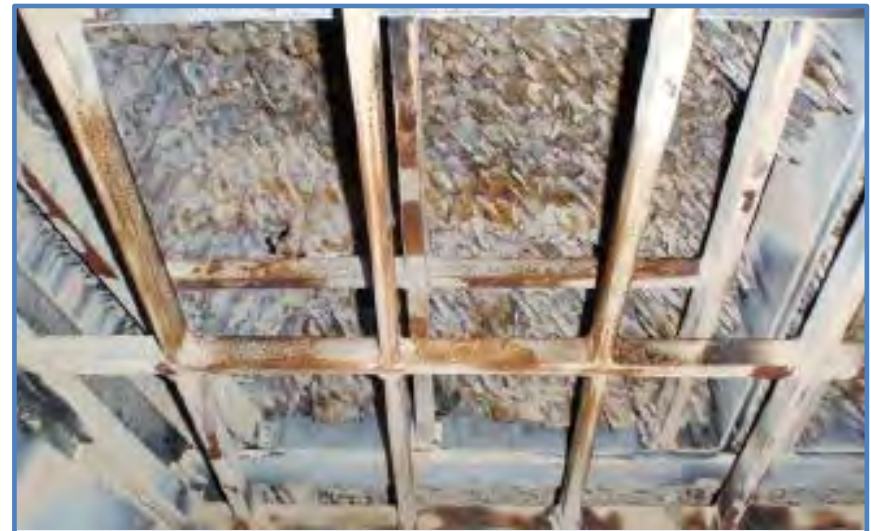
Brominated PAC - Upstream Injection
